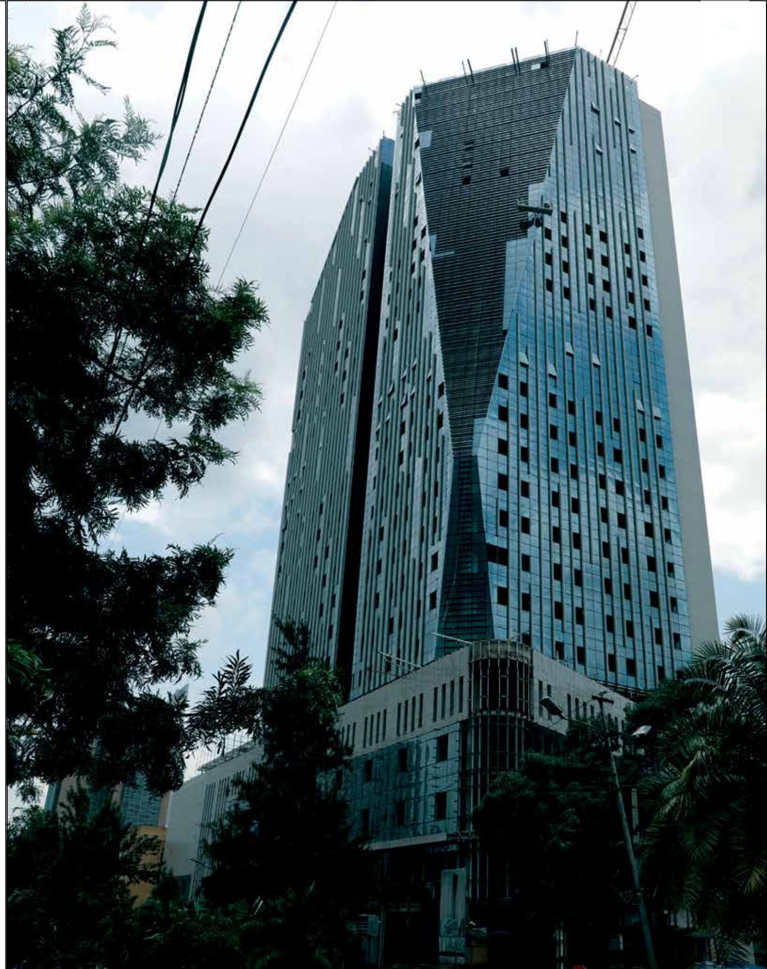
TSEDEY BANK HEAD OFFICE BUILDING UNDER CONSTRUCTION
